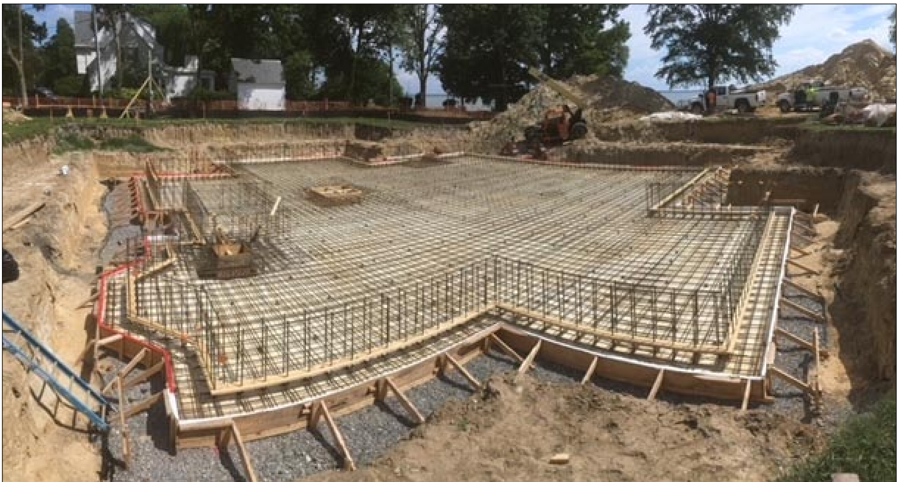
HRSD Generator Building — Image Property of A+ Concrete
