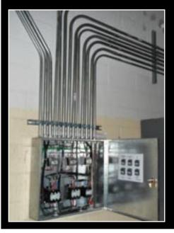
One of the key components of the Data Center is this Relay Panel, which enables all power to be disconnected in case of emergency...
